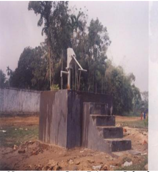
Narayanpasa Govt. Primary School, Moulvibazar
